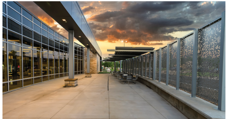
Base Maintenance Building Renovation, MMAC, OK FAA Mike Monroney Aeronautical Center A/E IDIQ
