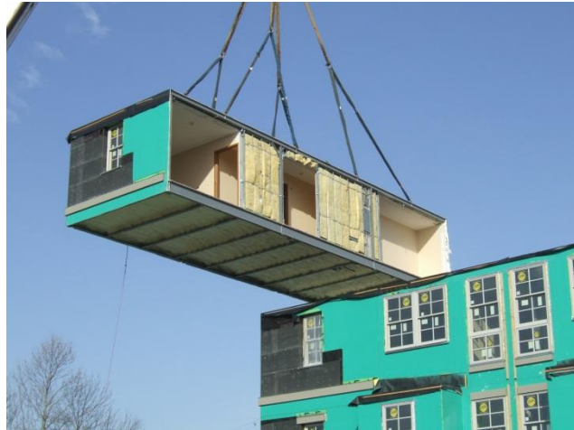
Figure 1 - Placement by crane, top pick
